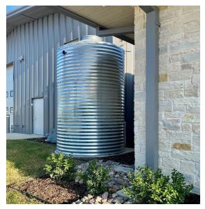
per year. These cisterns eliminate erosion from downspouts and improve water infiltration by 80%, reducing parking lot flooding and mosquito breeding. Included in the rainwater harvesting system is a rain garden that captures approximately an average of 34,750 gallons of rainwater per year from the downspouts off the overhang above the breezeway between the main office building and the shop building. The irrigated landscape areas support bees, butterflies, and hummingbirds.
